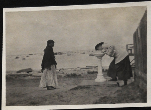
By the school-house, Neah Bay
